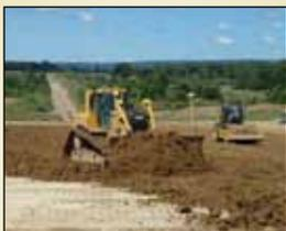
Clay barrier being placed over gas venting layers
