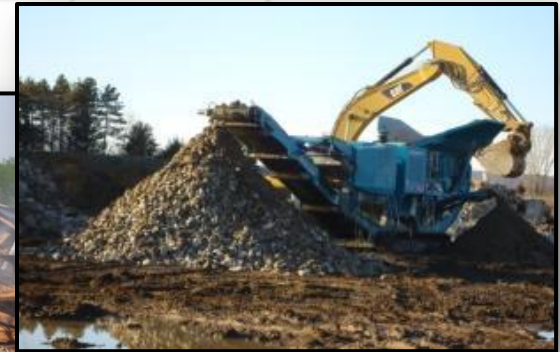
Crushing Concrete for Road Fill
