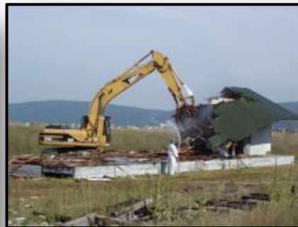
Contaminated Structure Removal
